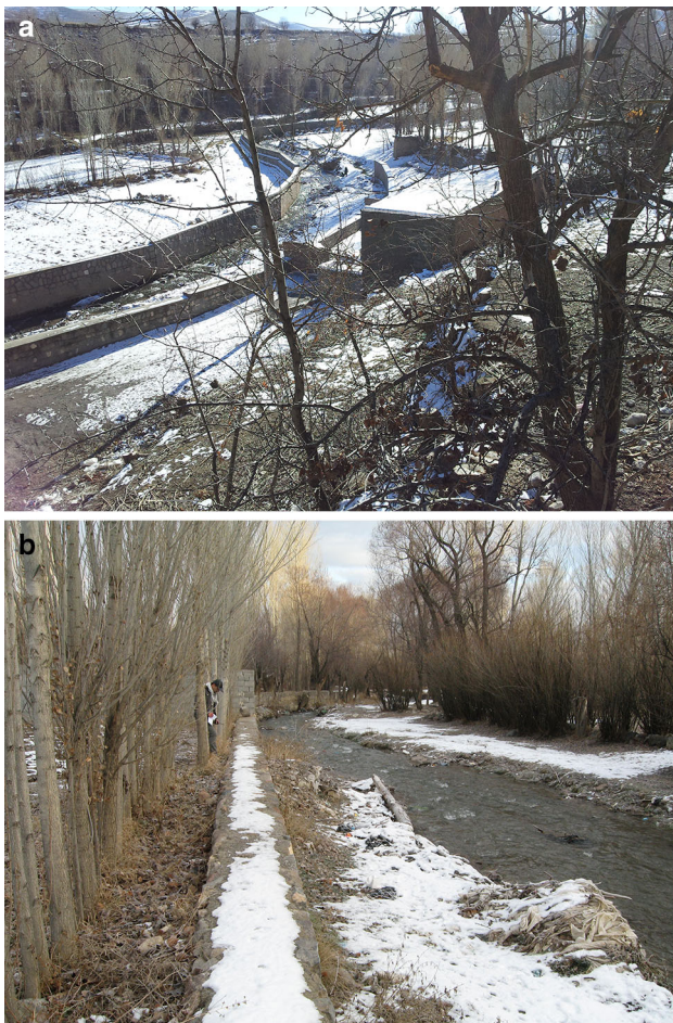
Fig. 3 Channelization (a) and bank protection structures (b) along the Lighvan River
