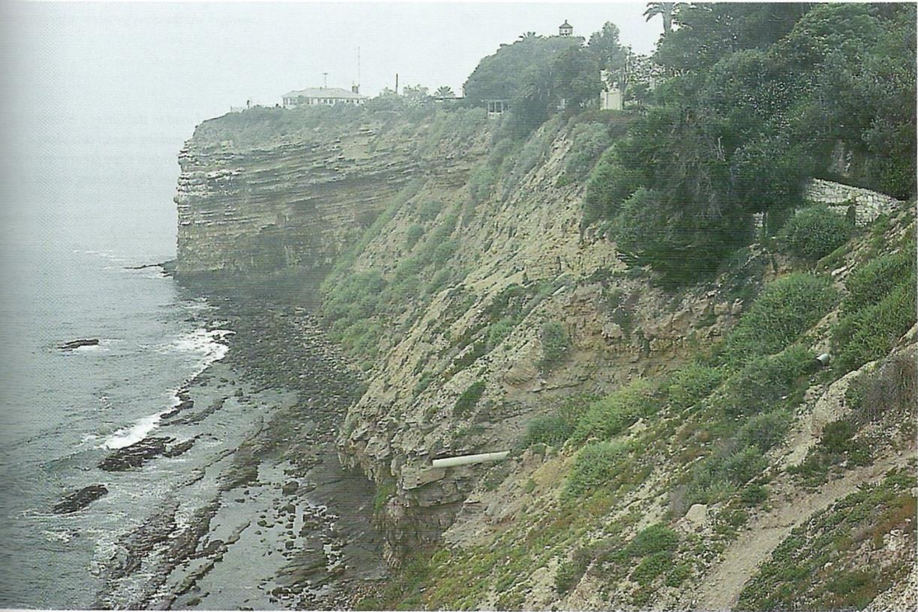
Figure 11.28 (a) Driving drainpipes that are perforated on one side into a hillside, with the perforated side up, can remove some subsurface water and help stabilize a hillside. (b) A drainpipe driven into the hillside at Point Fermin, California, helps remove subsurface water and stabilize the slope.
