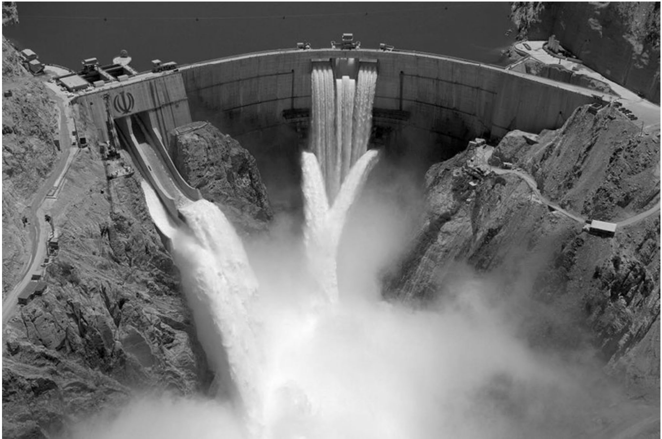
Fig. 1 Photograph of free-falling jets in Karun III dam in Iran
